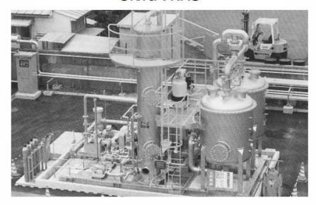
This plant collects valuable hydrocarbon resources efficiently and prevents air pollution caused by hydrocarbon vapor. Air pollution occurs during manufacturing, receiving and shipping in the oil refinery factories, oil tanks and oil chemical factories. The plant can be used to vaporize hydrocarbon like solvents such as gasoline, naphtha, and jet fuel.
