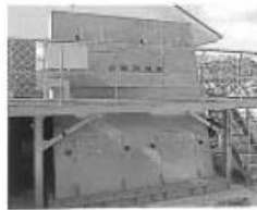
Screening equipment(rotary rake)
